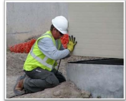
**(8)** Apply a row of Conseal base gasket to the slab, midway between the drilled holes and the traced outline of the building. Be sure that any Conseal butt joints are tight so that when they are compressed they form a continuous seal. In colder weather, warm up the Conseal to 75°F before applying to the slab.
