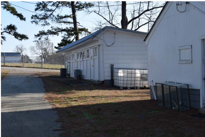
Shelters to be replaced
